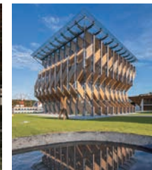
GREENable HIRUZEN(風の葉・水盤) ©Kawasumi-Kobayashi Kenji Photograph Office
